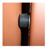
2) Retainer should be adjusted with temporary spacers against door in closed and latched position (See picture to the left.) If spacers are not present, the space between retainer and door face should be approximately 13/32".
