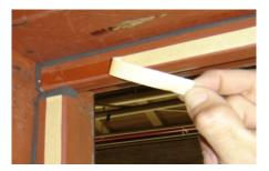
5) Remove the protective paper cover from the double-faced tape as well as any temporary bumpers from the retainer.
