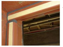
1) Retainers should be installed with sealing rubber completely sealed around 3 sides of the frame, as seen in the picture to the left.
