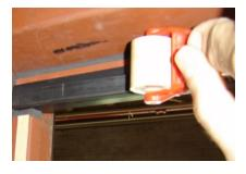
7) After seal has been completely installed, roll seal tightly with wall paper roller on similar tool. Repeat this rolling process over entire length 3 or 4 times.
