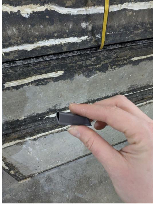
Figure 3 – “Bubble” gasket piece
