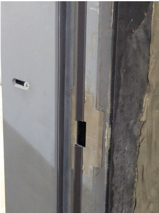
Figure 6 – Detail of “bubble” gaskets
