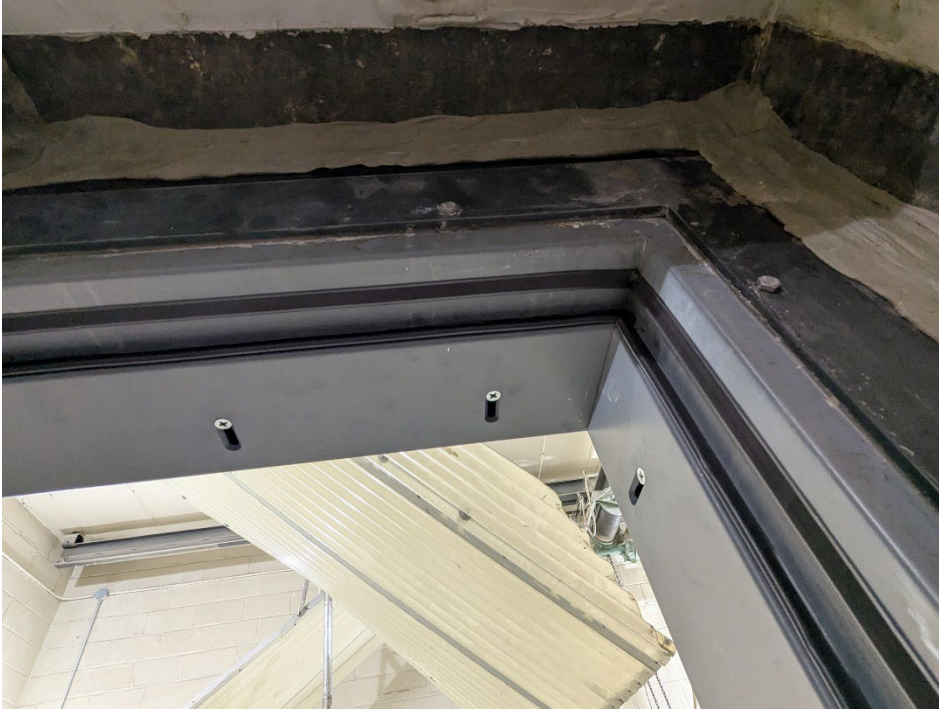
Figure 5 – “Bubble” gaskets installed along door frame and frame stops
