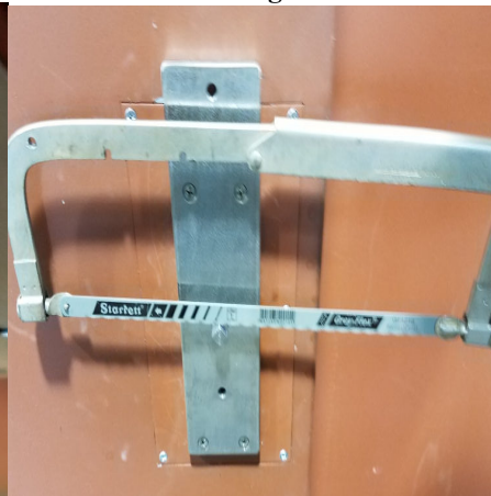
Mark and cut spindle.
