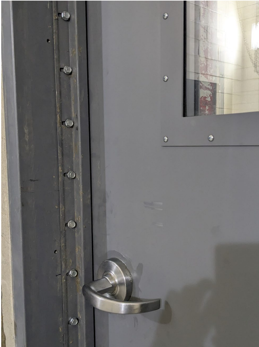
Figure 3 – H-seal retainers and seals installed
