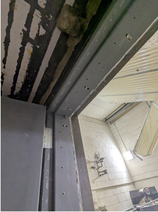
Figure 3 – Door stops installed in door frame
