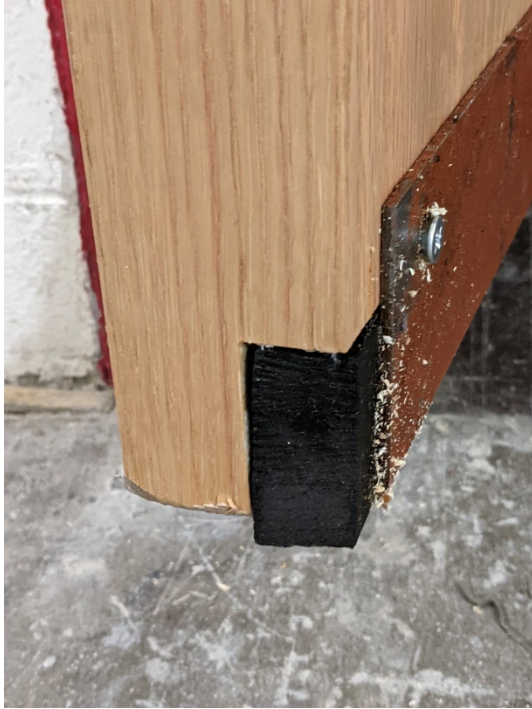
Figure 5 – Detail of door sweep configuration
