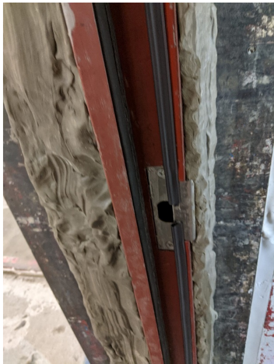
Figure 3 – Seals and gaskets at strike jamb
