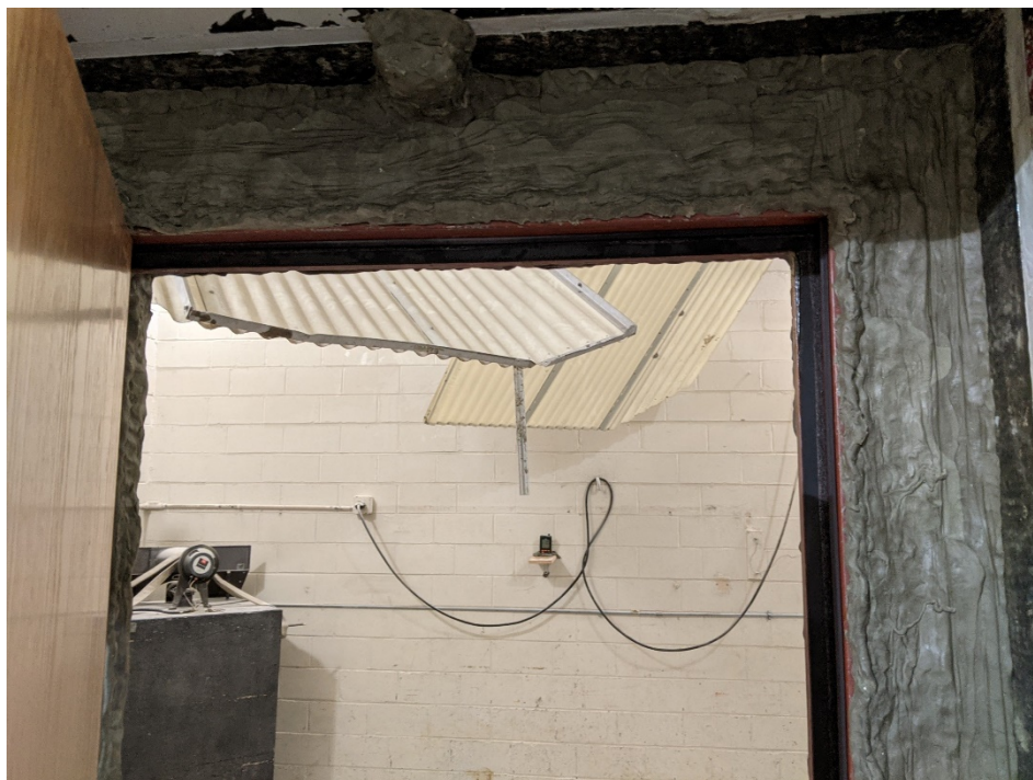
Figure 2 – Operation of specimen, as viewed from receive room; extent of perimeter mastic seal
