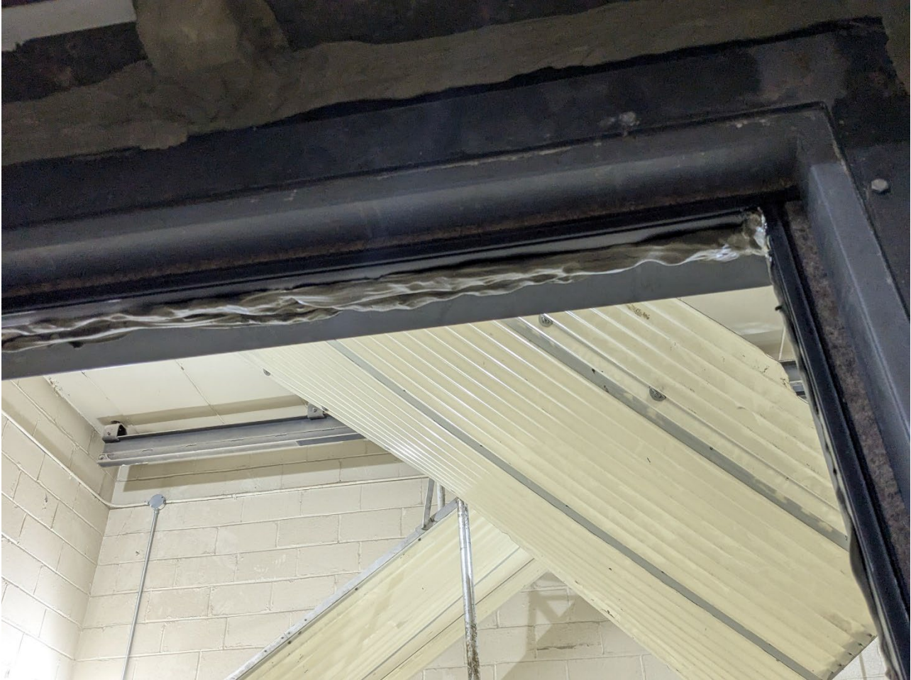
Figure 3 – Felt strips installed
