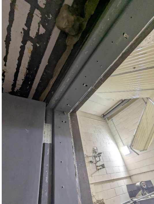
Figure 3 – Door stops installed in door frame
