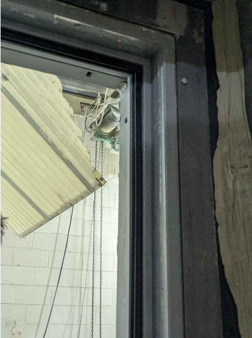
Figure 5 – Mag seal retainers with gaskets installed in door frame
