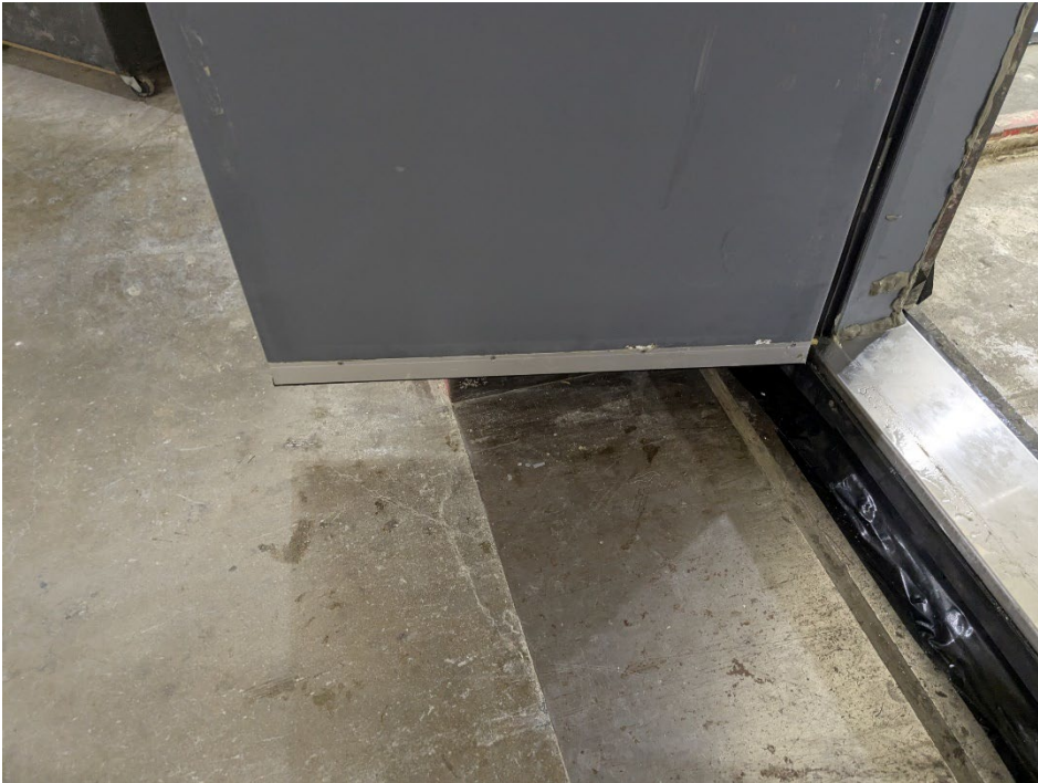
Figure 2 – Door bottom installed to leaf
