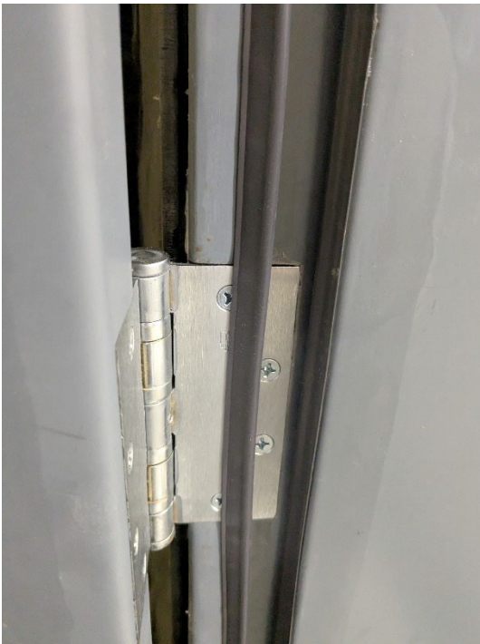
Figure 2 – Detail of installed door hinge (door seals in photo cut and adjusted prior to test)
