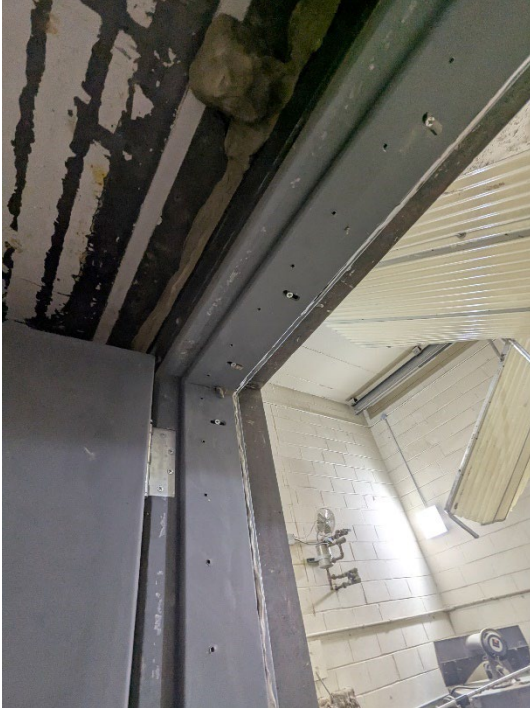
Figure 3 – Door stops installed in door frame
