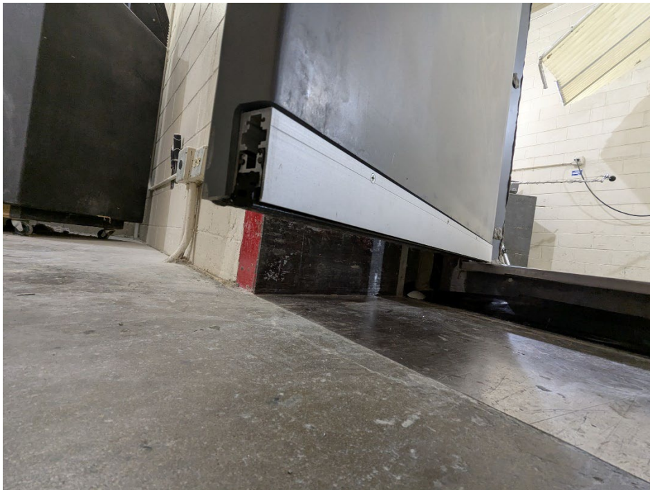
Figure 4 – Door bottom installed
